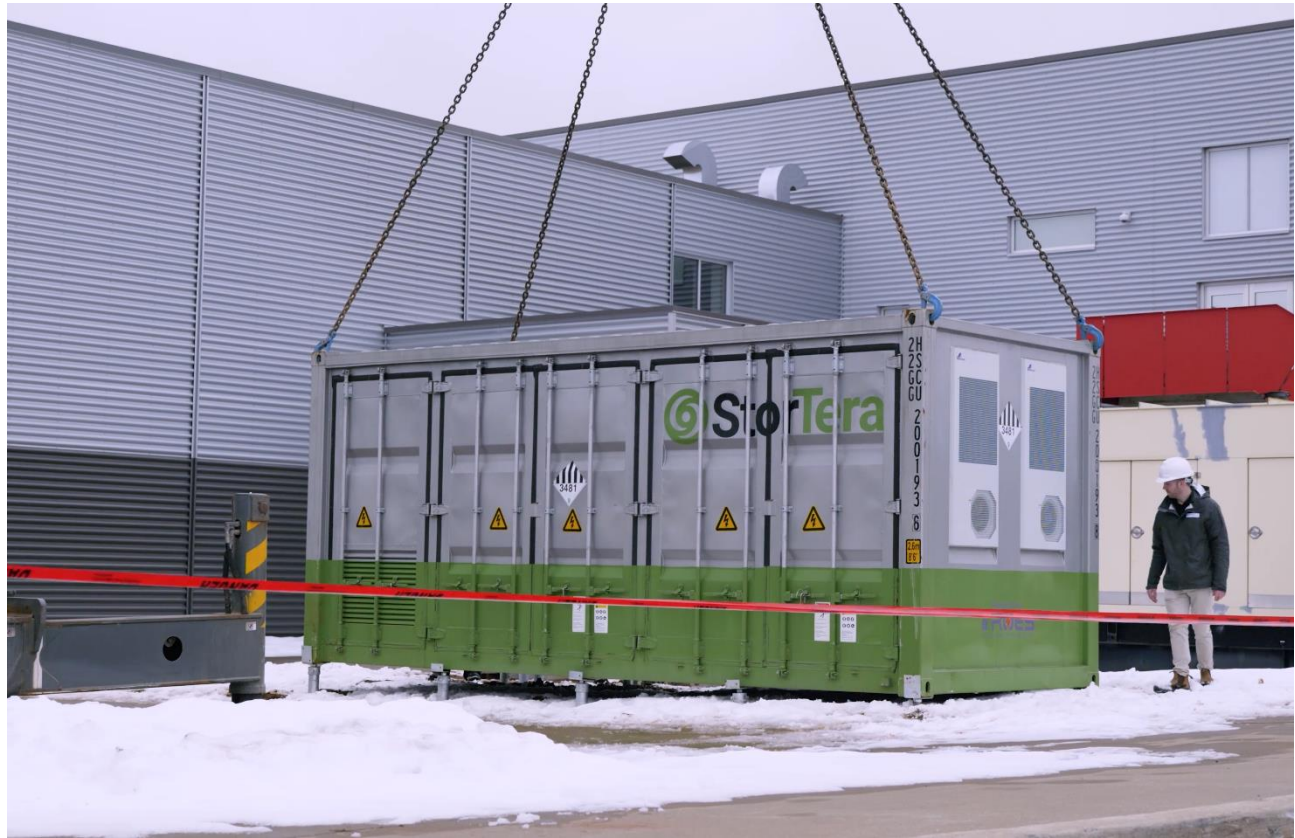
One of the StorTower commercial energy storage systems being installed in Berwick, Nova Scotia
