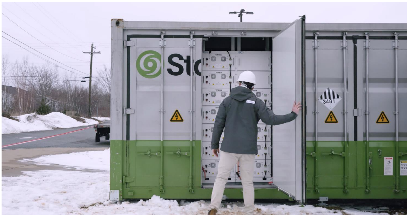
StorHub commercial system installation in Berwick, Nova Scotia
