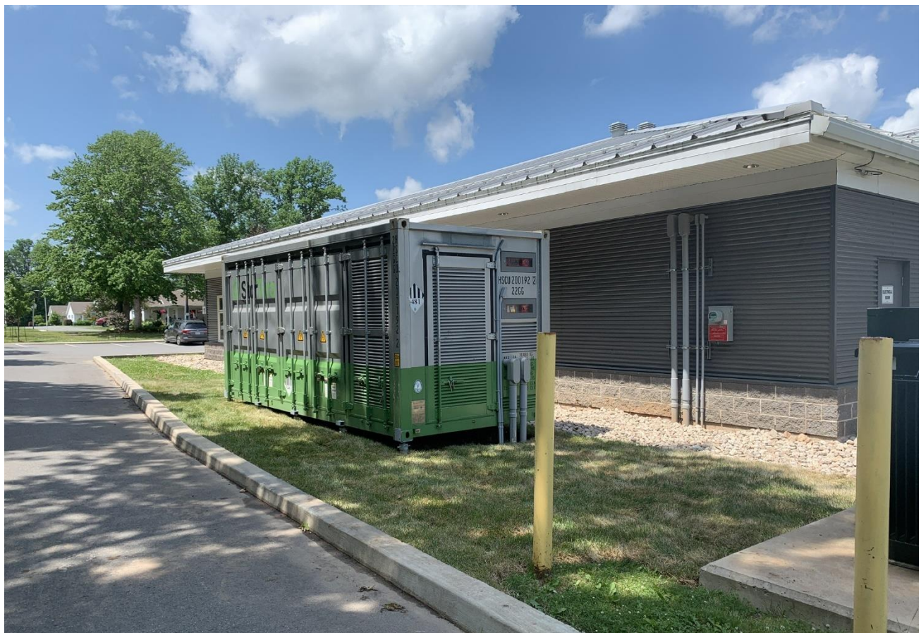
One of the StorHub commercial energy storage systems installed at the Town Hall in Berwick, Nova Scotia
